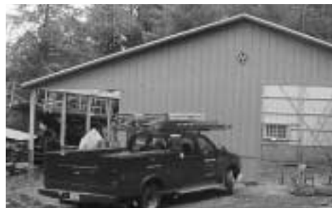
Morton Builders erecting our new Maintenance Building
