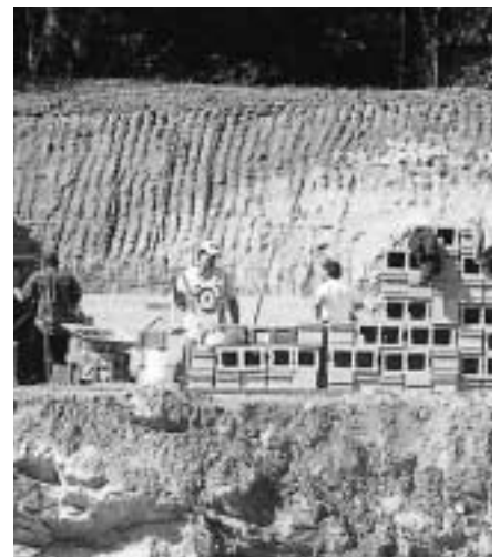
The concrete block is laid for Johnson Hall
