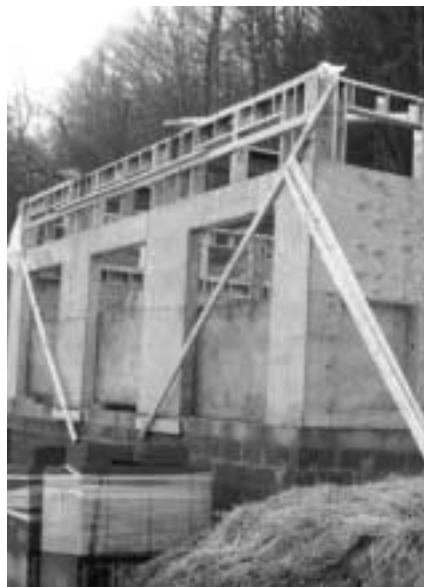
Work continues on Bishop Johnson Hall
