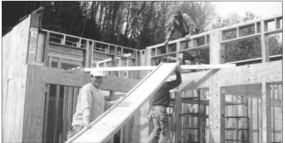
WORKERS LIFTING FLOOR BEAMS AT BISHOP JOHNSON HALL
