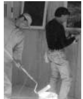
Left: Billy Kennedy and Dave Donovan applying stain to the outside of the hall.
